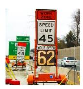
The Tollway's smart work zone system has shown proven success with the use of speed indicator boards to increase awareness of work zone speed limits, with studies demonstrating that speed decreased by as much as 14 mph when boards were used in work zones.
